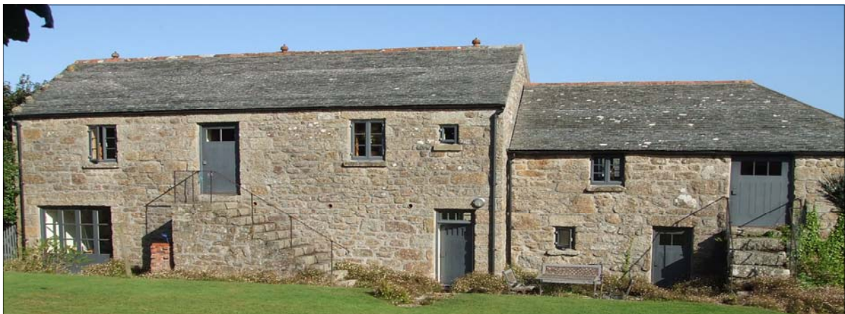
Example of a sensitive barn conversion for permanent residency
