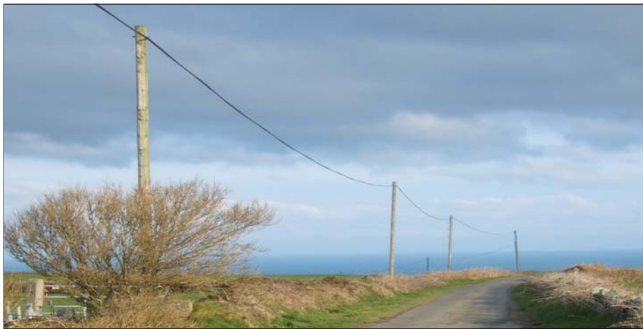
Unsightly overhead cables
